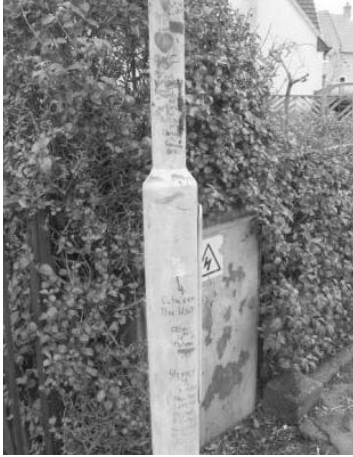
Graffiti on lamp post and utility box
