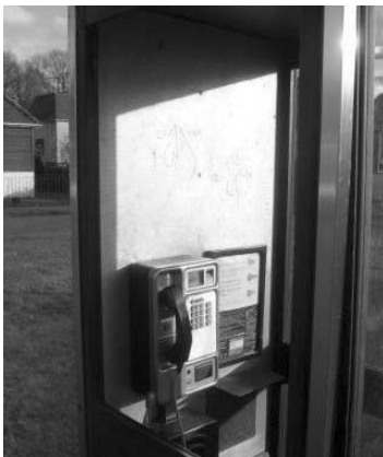
Telephone booth with missing glass panel (vandalism)
