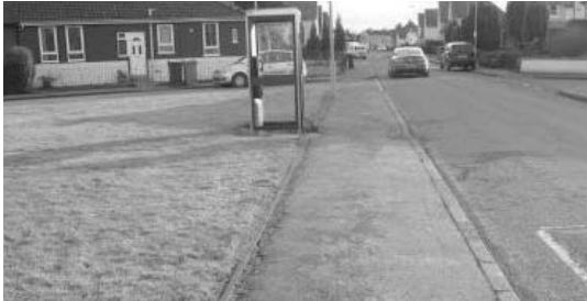
Pavement covered with grit
