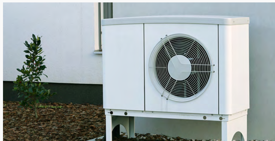
Heat pumps are a renewable technology that can be used to warm (or cool) buildings from thermal energy stored in air, ground or water. Image: Milan/AdobeStock.
