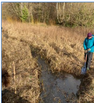
A volunteer digging a pool beside the stream that runs through marshland; by Friends of Easter Craiglockhart Hill
