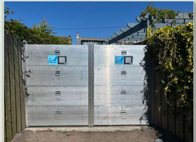
Installation of new flood gate Community Resilience
